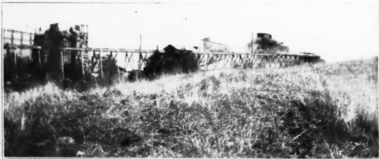
Flume for Carrying Sand and Water To Waste Area Shown in Illustration Above.
